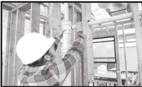
Plumbing Technology Apprenticeship Jonesboro
